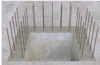
Post-installed rebar connections
