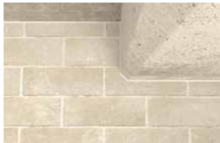
Construction joint application
