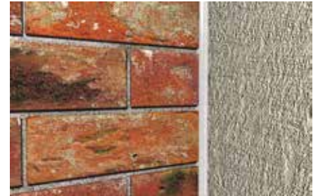
Vertical construction joint application
