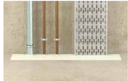
Mixed penetration through the floor
